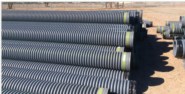
Stack pipe in a flat, clear area no higher than 6' (1.8 m). Use securing blocks to ensure pile does not collapse.
