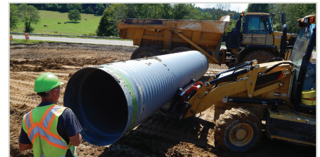
To prevent damage to the pipe, do not use forklift inside the pipe and avoid direct impacts. Do not drag or strike pipe ends against anything to avoid spigot or bell damage.
