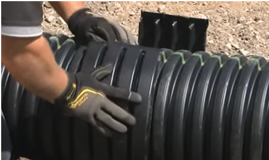
Split coupler being installed on N-12 plain end pipe.
