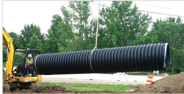
24"-30" (600-750 mm) diameter pipe requires a backhoe with one nylon sling.
