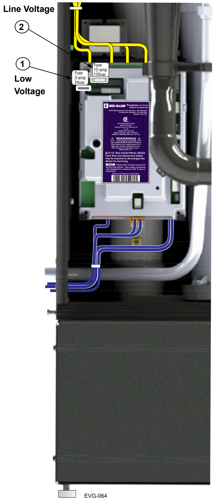
Figure 92 Control fuses
