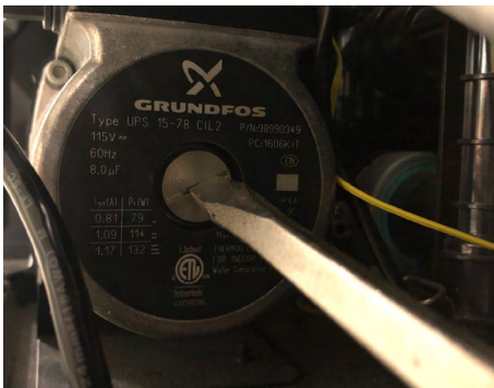
Figure 54 - Bleeding the Internal Pump
