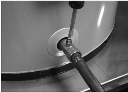
Draining the old water heater.
