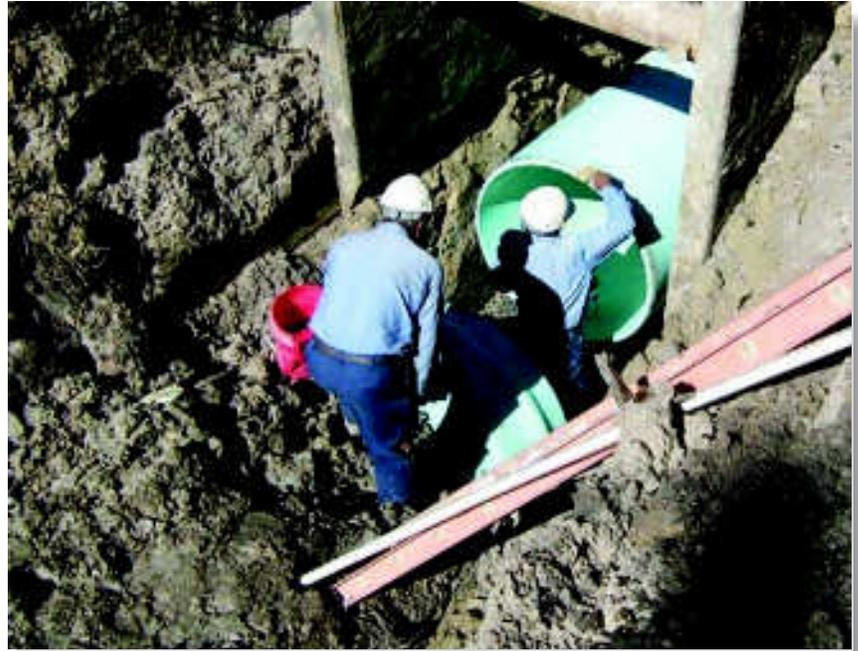
Each male end shall be beveled to facilitate joining and referencing marked for proper insertion depth. Diamond furnished lubricant is to be used in the joining process.
