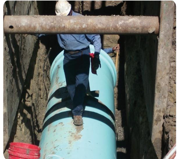
Sani-21 is supplied in 14 foot and 22 foot laying lengths.
