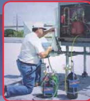
Purge and pressure test an A/C&R system
