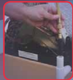
Clean out condensate drain lines with Sludge Blaster®
