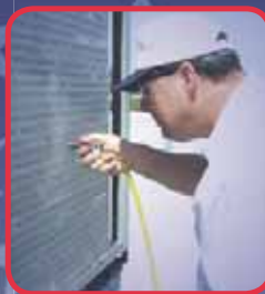
Blow off coils with Sludge Sucker® Blowgun
