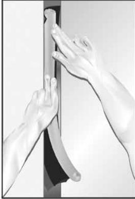
1. Clean all surfaces in joint area to remove loose debris, dirt, oil, wax, grease, old caulking, etc.
