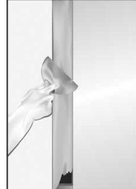
4. Trowel sealant to the desired finish. See tested UL systems for complete installation instructions.
