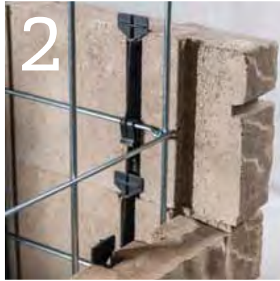
2 Use connector to attach Lafitt Tandem Veneers to grid
