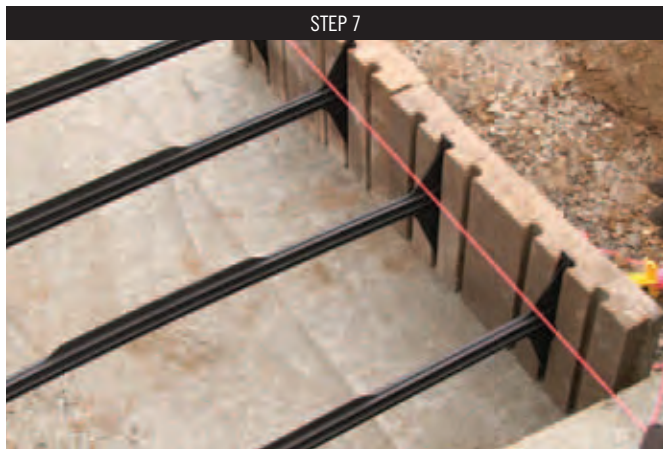
Run a string line from the back side of the front wall veneer to assure proper horizontal wall alignment.
