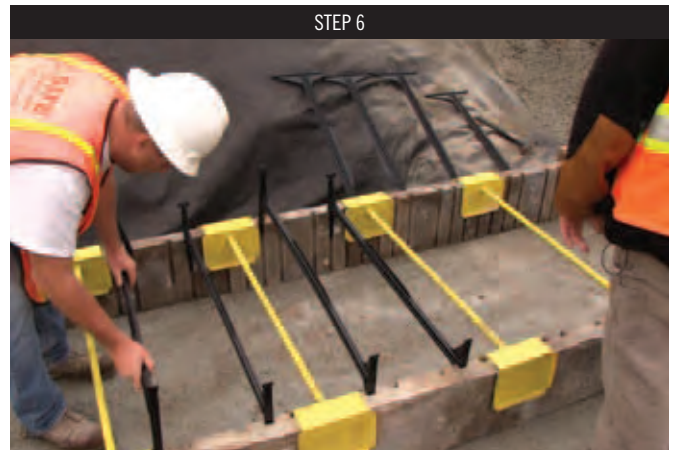
Insert the Mega-Tandem™ (MSRW) connecting members into the center dovetails to provide the structural support in the wall system.
