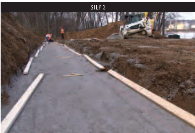
Forming up to pour a 2" unreinforced concrete overlay for setting the first course of Mega-Tandem™ (MSRW). A 6" crushed stone leveling pad is an option as well.
