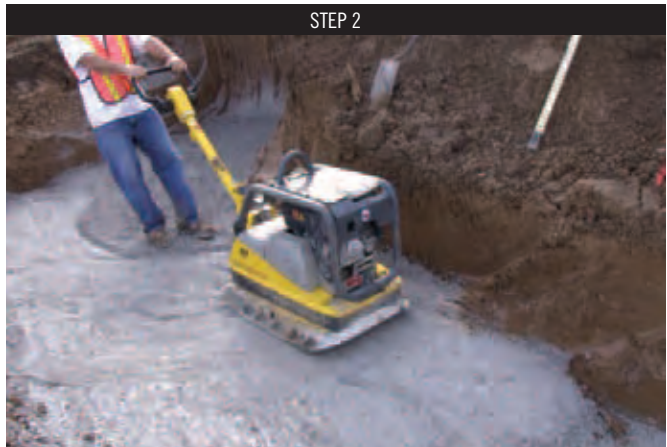
Compact the placed crushed stone to reach 95% standard proctor density.
