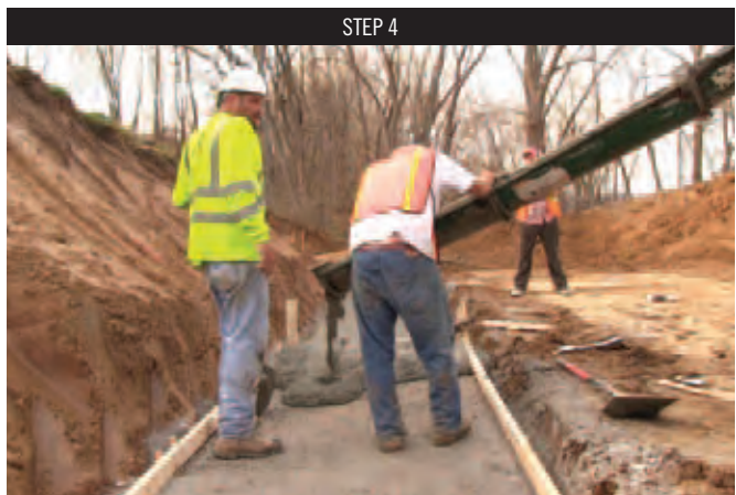
Pouring the leveling pad with a low psi concrete.
