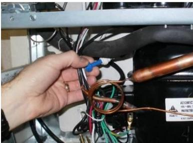
Next, insert end of tube into fitting.
