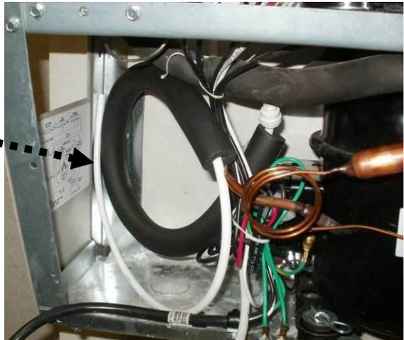
For split level “Versafiller ready” coolers, the tube to plumb in the Versafiller is packaged in the dummy unit or found inside the Bottle Filler.
