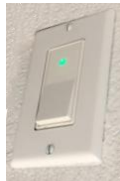
LED rocker switch installed in wall plate
