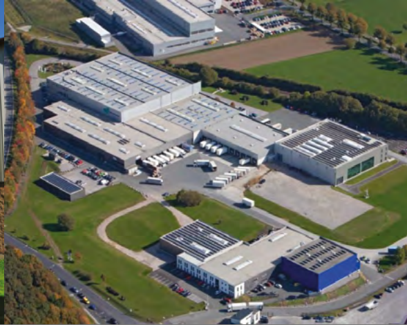
Centrotherm Systemtechnik GmbH Brilon, Germany
