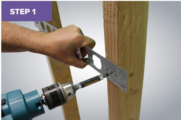
Install a **PEXRITE** (#103-18/103-26) bracket onto the front of wall studs.
