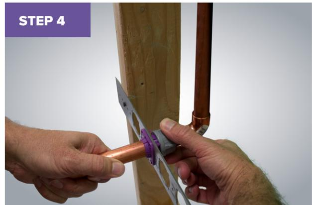
Slide a  $\frac{3}{4}$ " tube or bullet through the insert. Lock the tubing in position by tightening the grey nut clockwise, by hand.
