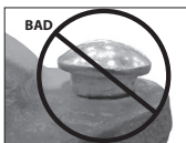
OVAL NECK OF BOLT NOT SEATED PROPERLY
