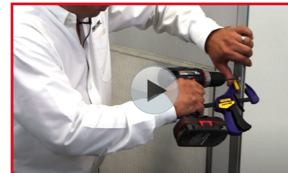
How-To Video: Installing a Screen Door Pet Grille
