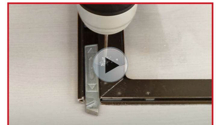
How-To Video: Replace slide bolts in a storm window
