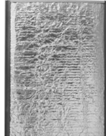
All panels in the evaporator section of the unit have cleanable foil-faced insulation. All edges are either captured or sealed to ensure no insulation fibers get into the airstream.
