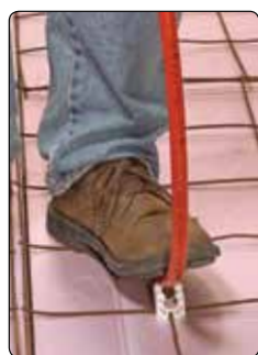
Protective plastic-to-plastic PEX connections
