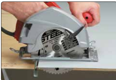
Standing Seam Metal Roofing
