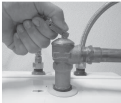
Figure 31 - T&P Relief Valve
