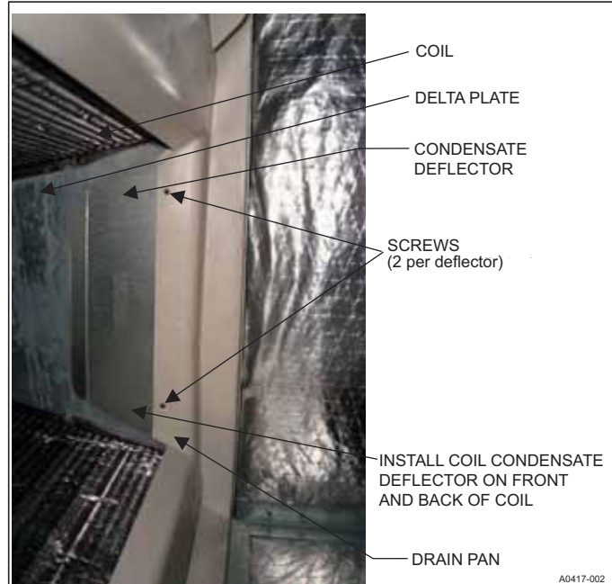
FIGURE 6: Coil Condensate Deflector Installation
