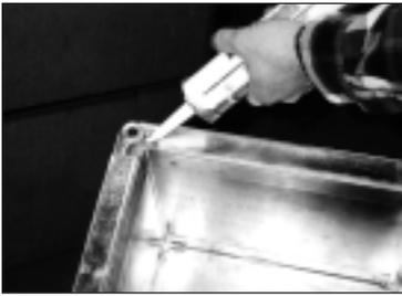
1. Cut, assemble and attach Ductmate frames to ductwork according to the normal procedures listed in steps 1 - 12 of the assembly instructions.
