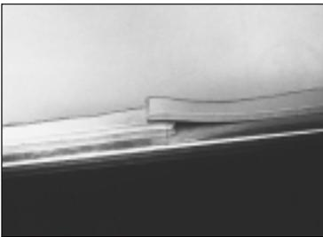
15. Apply 440 gasket completely around Ductmate frame to the beginning point. Where gasket meets overlay about 3/8".
