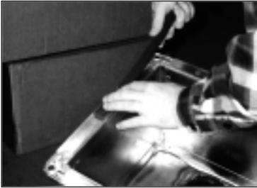
2. Wipe off the face of the Ductmate flanges and corners with a dry cloth where gasketing and sealant will be applied
