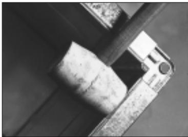
7. If the duct corner or the Pittsburgh lock gets caught under the Ductmate corner, tap the frame outwards to allow the duct corner to slide past the Ductmate corner piece. **THIS IS VERY IMPORTANT!**
