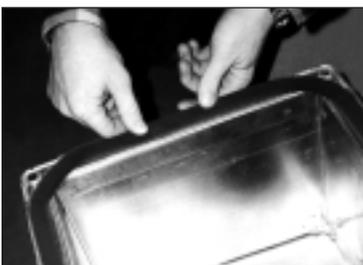
4. Apply the Ductmate Neoprene gasket around the perimeter of one duct section of the connection. Start gasketing half way between corners, favoring the outside edge of the Ductmate flange. Apply gasketing in an arc at all four corners, making sure to cover the key points shown. Butt the end of the gasket tight against the starting point.
