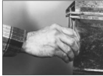
5. Align duct sections to be connected. Bolt duct sections together at all four corners using 1" x 3/8" bolts for the Ductmate 35 system and 1" x 5/16" bolts for the Ductmate 25 Systems. Do not use the Ductmate "no bolt clips" for removable duct applications.
