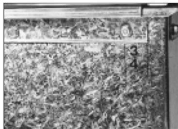
11. It is essential that the frame angle is fastened to the duct within  $\frac{3}{4}$ " of the end of the angle at each corner.
