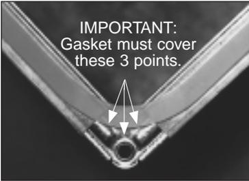
14. Position 440 Gasket in an arc so that it covers the three points in the duct corner. *Gasket must cover all three points.* Some gasket will protrude into the airstream. Press gasket firmly into contact with the raw edge of the duct corner and Ductmate corner assembly. Ductmate 440 is the preferred gasket. Refer to procedures on the back of the brochure for applications using Ductmate Neoprene Gasket.
