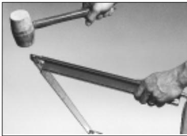
5. Now complete the frame by seating the corner pieces into the Ductmate angle.
