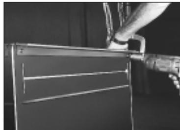
10. Work in one direction around duct when seating the frame. Fasten in sequence as you go. Do not fasten angle at corners first, it can cause seating problems.
