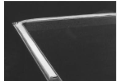
13. Systems '25' and '35' use 5/8" Ductmate 440 Gasket Tape. Start applying halfway between duct corners. Position in center of Ductmate angle as in photo.
