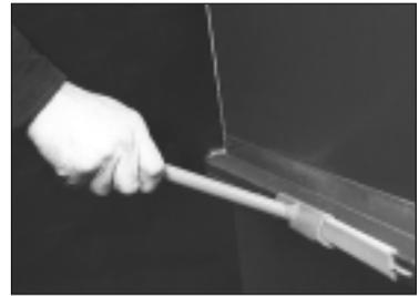
21. Ductmate 25/35 cleat can be snapped-on with the Cleater I Tool or with the Cleater II where space is restricted.
