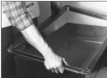
6. Start completed Ductmate frame at corner of duct.
