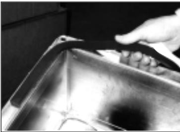
3. Apply Ductmate PROseal water based sealant to all eight corners of the connection as shown. Be sure to cover the gaps between the corner and ductwall. Allow sealant to dry prior to application of the gasket.
