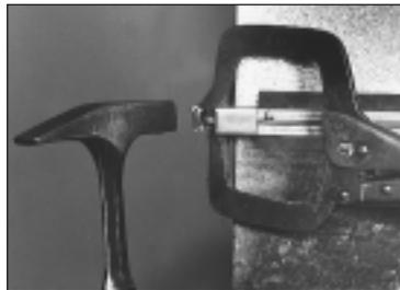
19. Slide corner clips onto the Ductmate 25/35 joined corner pieces. Tap with hammer until rear tab clicks into notch on corner pieces and locks in for a permanent connection.
