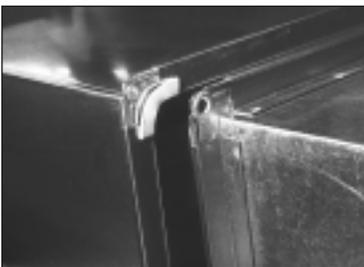
16. On the mating Ductmate frame apply 440 gasket only to the corners as in photo (approximately 3" per corner). The same 3 point application requirements apply as in photo 14.
