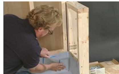
2. Fold corners and fasten upturns to studs.
