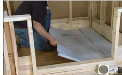
1. Install Chloraloy allowing for upturns - exact measurements not required.
