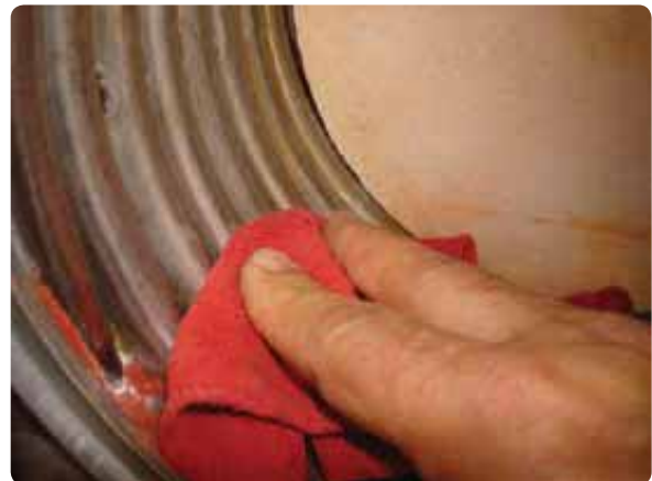
Figure 148 Cleaning the heat exchanger
