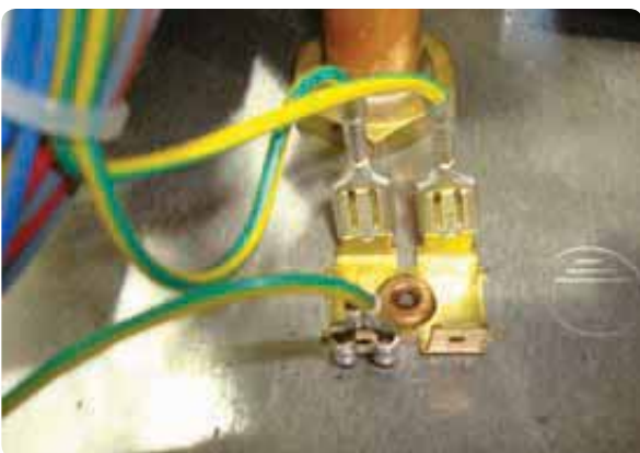
Figure 139 Ignition electrode grounding
