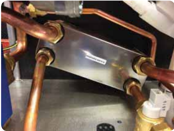
Figure 156 Removal of flat plate heat exchanger by loosening the four fittings. Combi-155
