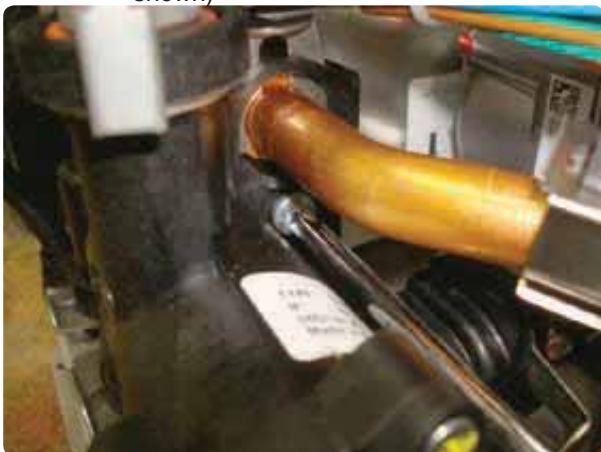
Figure 153 Removal of flat plate heat exchanger (screw on left side) (Combi Only 80/120 shown)
