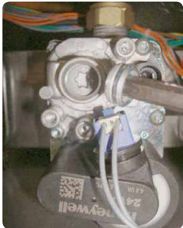
Figure 104 Remove T-40 cover cap with supplied Torx wrench for adjustment
