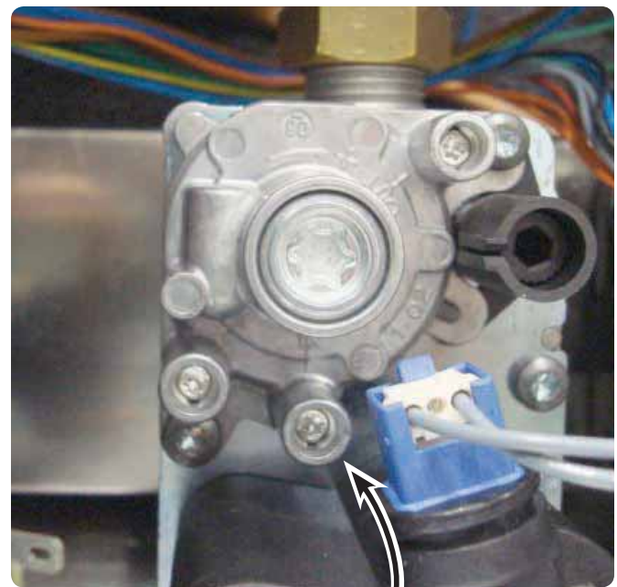
Figure 60 Inlet test port on gas valve
