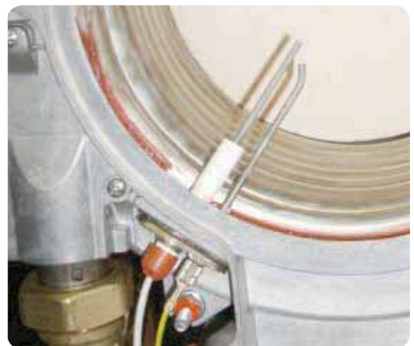
Figure 137 Inspecting ignition electrode
