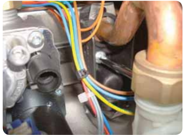
Figure 158 Removal of flat plate heat exchanger (screw on right side) (Combi Only 80/120 shown).
