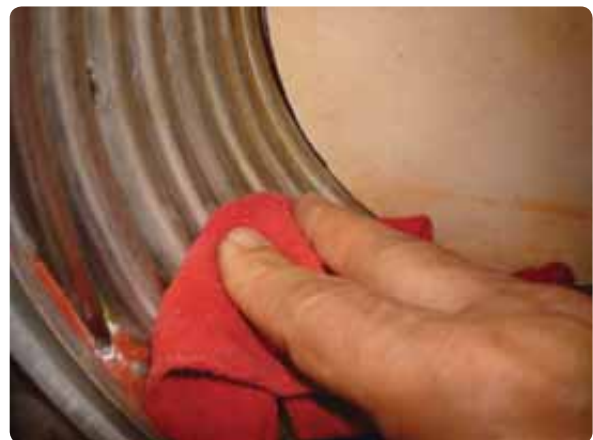
Figure 152 Cleaning the heat exchanger
