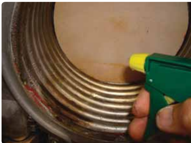
Figure 150 Cleaning the heat exchanger
