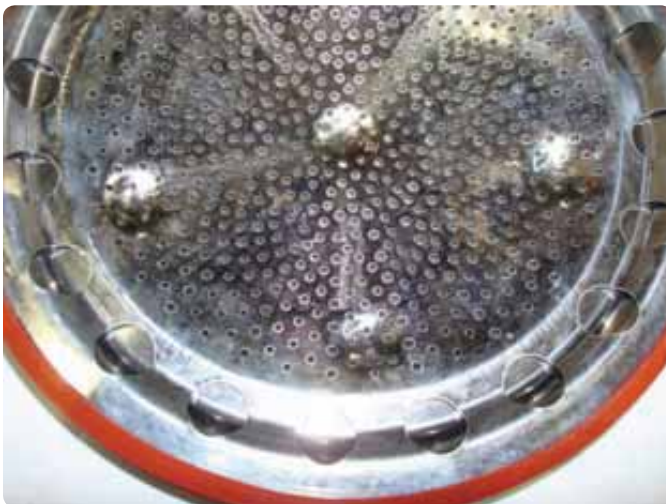
Figure 147 Inspecting interior and cleaning the burner
