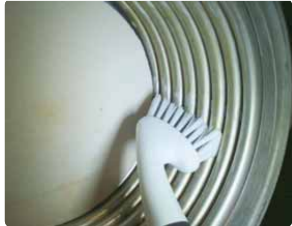
Figure 151 Cleaning the heat exchanger
