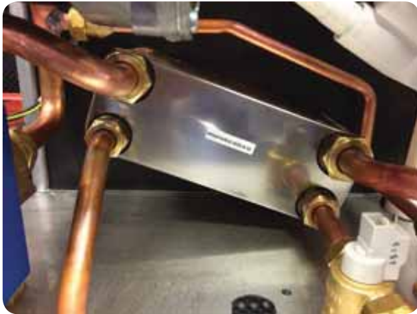
Figure 160 Removal of flat plate heat exchanger by loosening the four fittings. Combi-155
