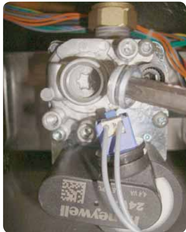
Figure 108 Remove T-40 cover cap with supplied Torx wrench for adjustment
