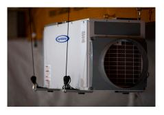
6 Adjust the height of the hanging bracket by either pulling on the cable or inserting the Gripple key to release tension.
