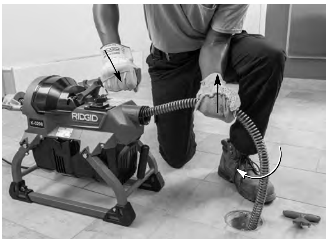
Figure 14A – Clutch Engaged, Cable Rotating, Pulling Cable Out of Drain
