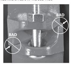
IMPROPERLY ASSEMBLED JOINT
