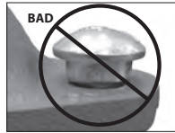
OVAL NECK OF BOLT NOT SEATED PROPERLY
