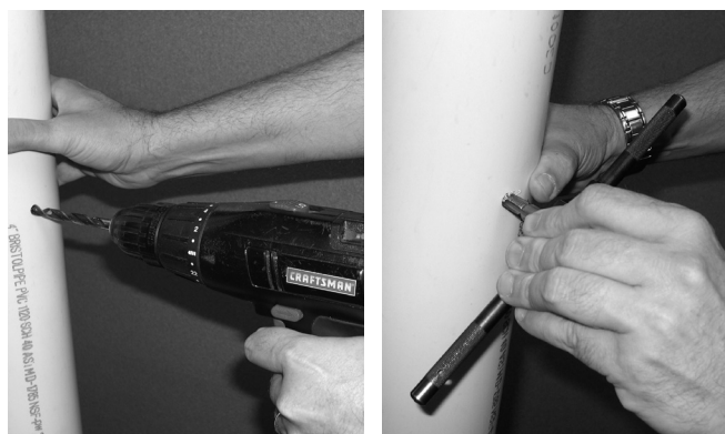
Figure 9.1: Drill and Tap Combustion Test Port
