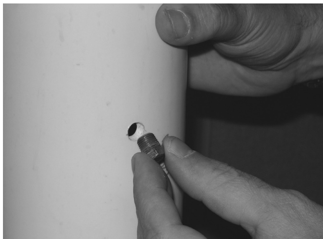
Figure 9.3: Insert Pipe Plug into Test Port
