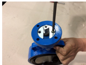
11. With a rubber mallet, tap the upper stem the remainder of the way into the stem. Secure the retainer plate with flat head counter-sunk screws.
