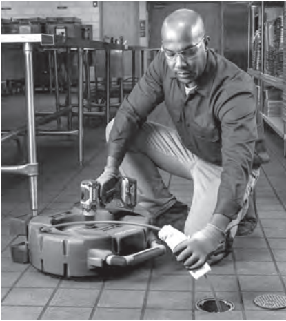
Figure 13 – Applying Lubricant to the Cable Sheath
