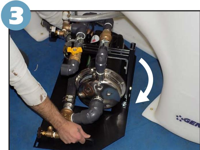
3 Slide the right side of pump assembly out first using the handles on the sides of the base plate.
