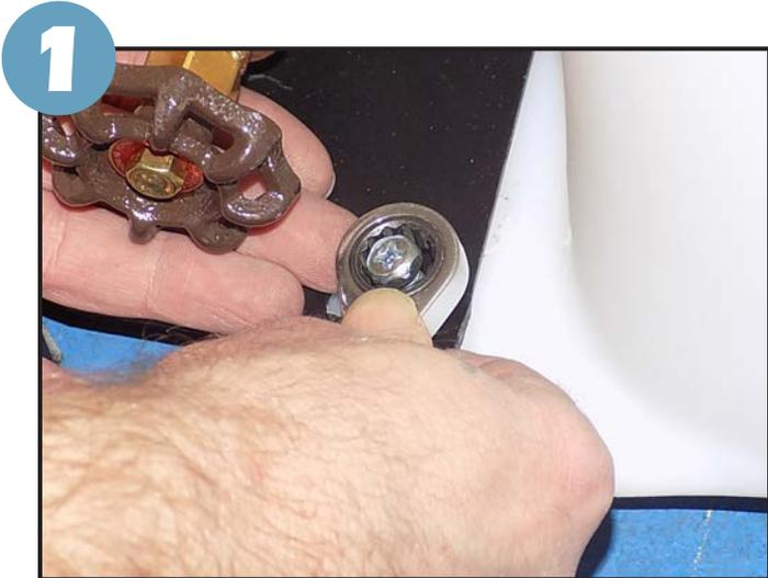
1 Remove the bolts on both sides of base plate.
