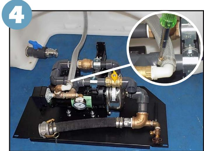
4 Continue to pull the pump assembly out by the base plate handles & disconnect the test hose.
