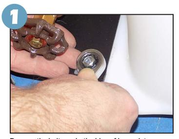
Remove the bolts on both sides of base plate.
