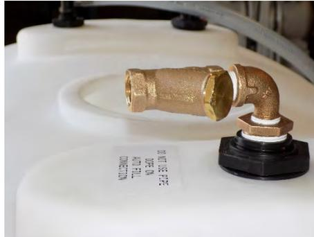
When installing Y-Strainer piping manifold DO NOT use pipe dope on any connection point leading up to the autofill bulkhead.
