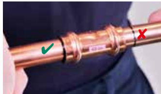
8. Insert the tube fully into the fitting. Ensure tube is fully inserted prior to pressing
