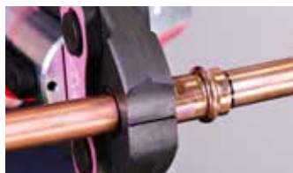
2. Complete the joint with the approved tool. Press once only
