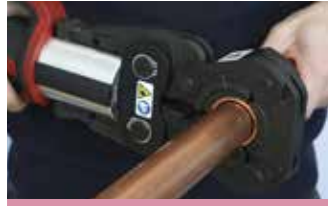
3. Complete the joint with the press tool
