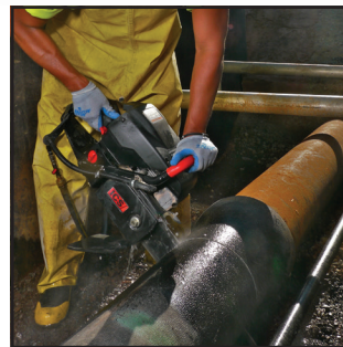
Safer to cut ductile iron
