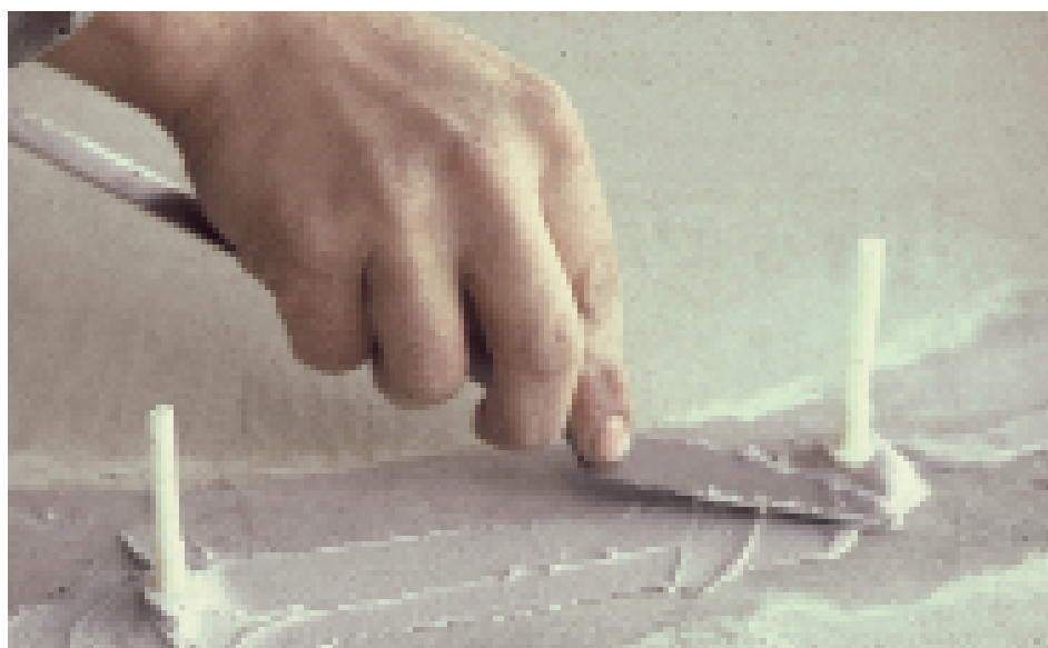
Capping crack with bulk CP-1400
