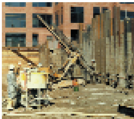
Grout used for Tie Back application
