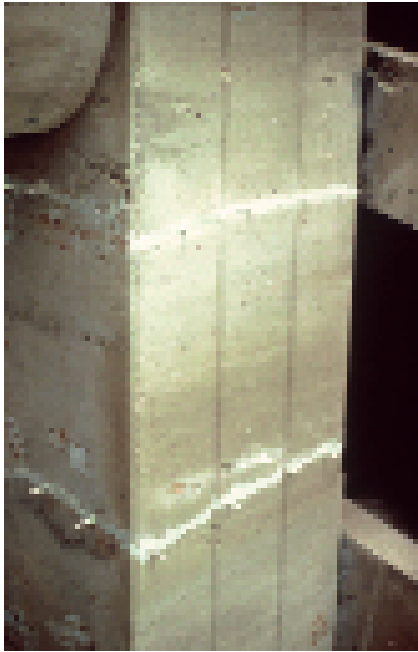
Here, a column is capped and ready for injection.
