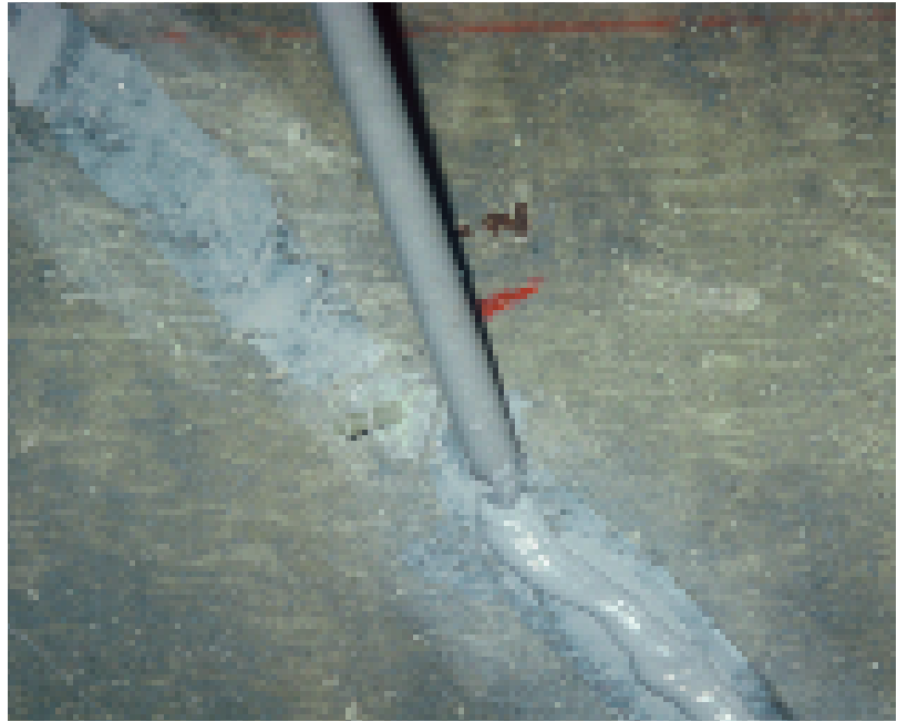
Capping a crack with CG-300.
