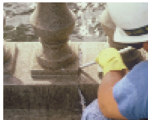
CG300 being applied to cap the crack.
