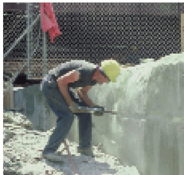
The capping material is ground off after the crack is repaired.
