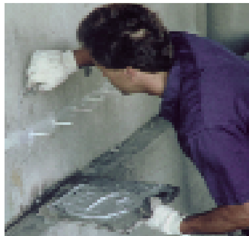
Capping crack with bulk CP-1400
