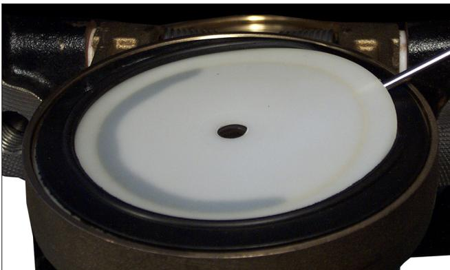
4. Pry the edge of the old seal washer from inside the clapper seal, as shown above.
