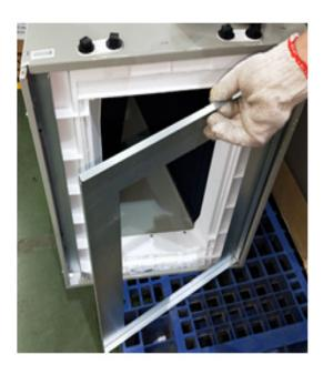
**STEP 5** - Reinstall the lower front panel using the screws removed in Step 1.
