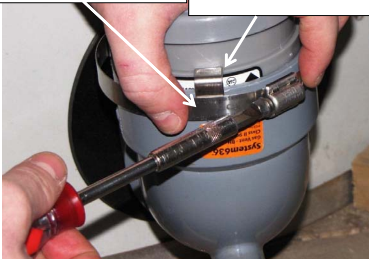
Flue Clamp Brackets on PVC Adapter Shoulder
