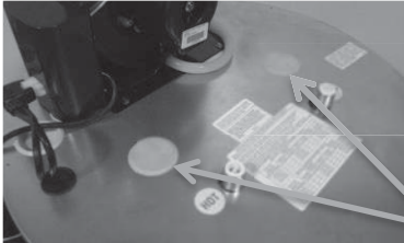
Anodes are located under caps
