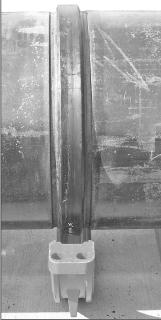
**4. JOIN PIPE ENDS:** Align and bring the two pipe ends together. Slide the gasket into position, and center it between the groove in each pipe end or AGS Vic-Ring.
