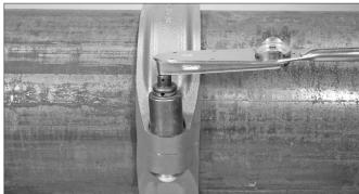
7. TIGHTEN NUTS: Tighten the nuts evenly by alternating sides. Make sure the housings' keys engage the groove completely in each pipe end or AGS Vic-Ring. Continue to tighten the nuts evenly by alternating sides until metal-to-metal bolt pad contact AND the specified torque value are achieved. Refer to the "Required Assembly Torques" table on this page.
