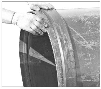
**3. POSITION GASKET:** Position the gasket over the pipe end or AGS Vic-Ring. Make sure the gasket does not overhang the pipe end or AGS Vic-Ring.
