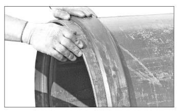
**3. POSITION GASKET:** Position the gasket over the pipe end or AGS Vic-Ring. Make sure the gasket does not overhang the pipe end or AGS Vic-Ring.
