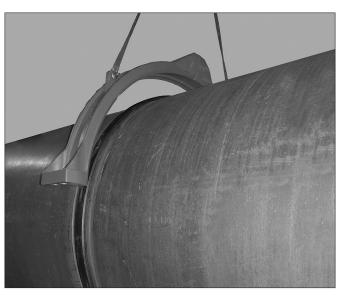
**7. MOVE UPPER SEGMENT ASSEMBLY INTO POSITION:** Using a strapping method, similar to the one shown in the above photo, install the upper segment assembly over the gasket. Make sure the housings' keys engage the groove completely in each pipe end or AGS Vic-Ring.
