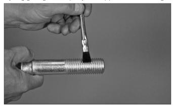
**8. LUBRICATE BOLT THREADS:** Apply a thin coat of Victaulic lubricant or silicone lubricant to the bolt threads. **NOTE:** If stainless steel bolts and nuts are special ordered, apply an anti-seize compound to the bolt threads.
