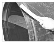
**1b.** Clean the outside surface of the pipe, from the groove to the pipe end, to remove all oil, grease, loose paint, and dirt.
