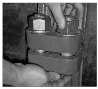
**6a. INSTALL FLAT WASHERS/NUTS:** Install a flat washer (supplied with the coupling) onto the end of each bolt, and thread a nut fingertight onto each bolt. **NOTE:** Make sure the oval neck of each bolt seats properly in the bolt hole.
