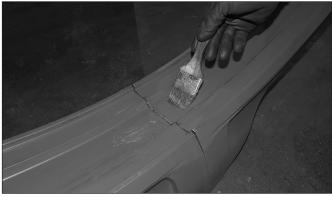
**4. CHECK GASKET AND LUBRICATE:** Check the gasket to make sure it is suitable for the intended service. The color code identifies the gasket grade. Apply a thin coat of Victaulic lubricant or silicone lubricant to the gasket lips, gasket exterior, and the interior surface of the coupling housings. Apply extra lubricant to the bolt pad mating areas, as shown.
