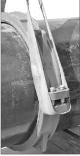
**6. INSTALL HOUSINGS:** Using a strapping method, similar to the one shown in the photos above with the bolts installed in the bolt holes, install the housings over the gasket. Make sure the housings' keys engage the groove completely in each pipe end or AGS Vic-Ring.
