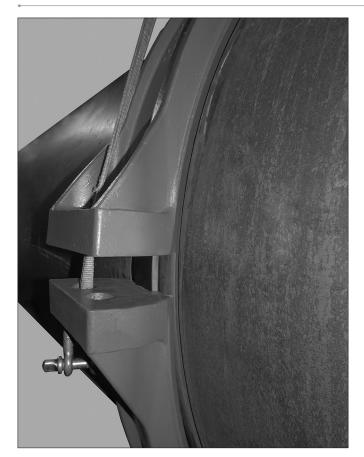
**9. RAISE THE LOWER SEGMENT ASSEMBLY INTO POSITION:** Using a strapping method, similar to the one shown in the above photo, raise the lower segment assembly. Make sure the housings' keys engage the groove completely in each pipe end or AGS Vic-Ring.
