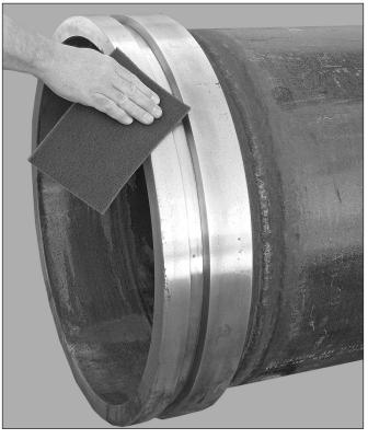
**1b.** Clean the outside surface of the Vic-Rings to remove dirt and other foreign material.
