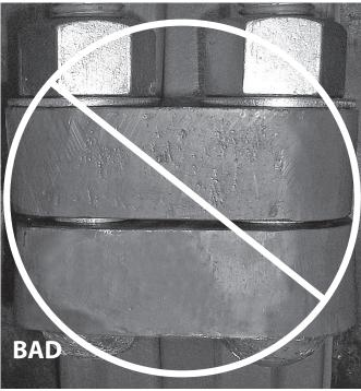
**8.** Visually inspect the bolt pads at each joint to ensure metal-to-metal contact is achieved across the entire bolt pad section.
