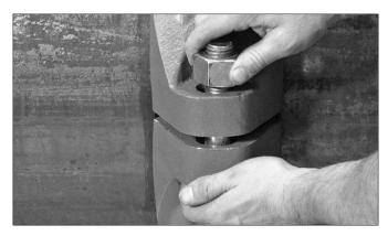
**6. INSTALL HOUSINGS:** Install the housings over the gasket. Make sure the housings' keys engage the groove completely in each pipe end or AGS Vic-Ring. Support the segments while preparing to install the bolts and nuts.
