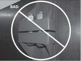
11. Visually inspect the bolt pads at each joint to ensure metal-to-metal contact is achieved across the entire bolt pad section.
