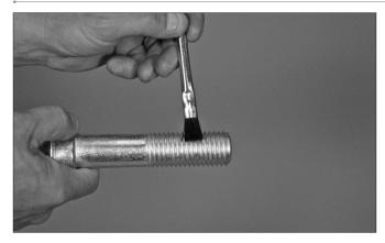
**5. LUBRICATE BOLT THREADS:** Apply a thin coat of Victaulic lubricant or silicone lubricant to the bolt threads. **NOTE:** If stainless steel bolts and nuts are special ordered, apply an anti-seize compound to the bolt threads.
