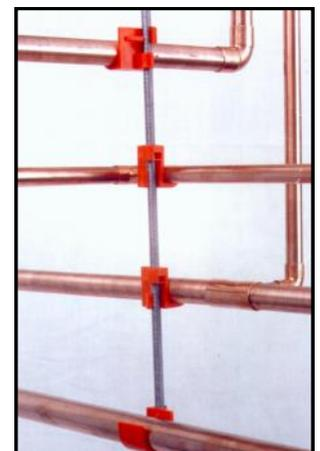
Place Hanger around rod as shown. Then twist until vertical and locked into place. Snap tubing into place.
