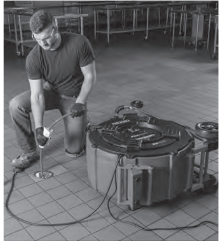
Figure 9 – Applying Lubricant to the Cable Sheath
