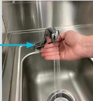
**STEP 8** Once all the air is purged from the system, and there's a solid flow of water from the faucet, turn off the faucet by removing hand from sensor motion area.
