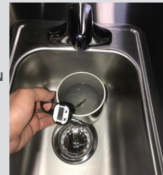
**STEP 12** If temperature needs further adjustment, adjust the mixing valve inside the cabinet.
