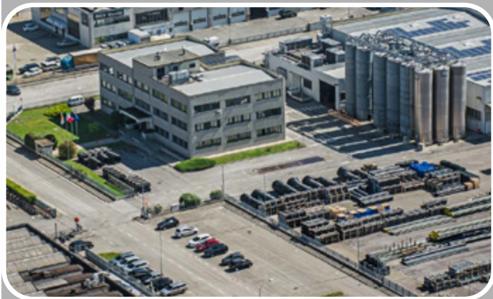
Production Facility - Castel Guelfo di Bologna (BO)
