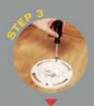
Secure toilet flange to floor with fasteners.
