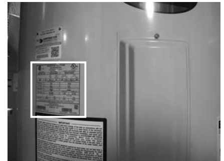
Figure 23 - The water heater’s electrical requirements can be determined from the data plate.
