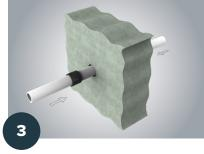
Slide wrap strips along the pipe and into the annular space as shown.
