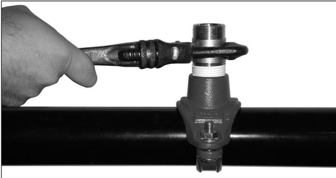
1. Apply pipe joint compound or PTFE thread sealant tape to the tapered threads of the adapter nipple, in accordance with the pipe joint compound or tape manufacturer's instructions. Using a pipe wrench, tighten the adapter nipple into the sprinkler piping.
