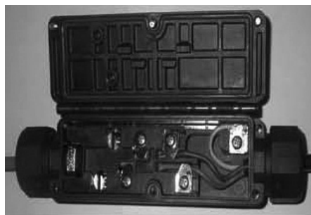
Figure 3-26: Secure terminals with screws
